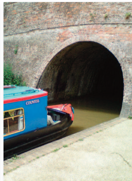
Entrance to The Blisworth Tunnel at Stoke Bruerne
